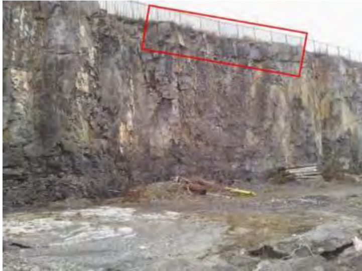
Figure 5.2: Wedge failure in the upper bench
